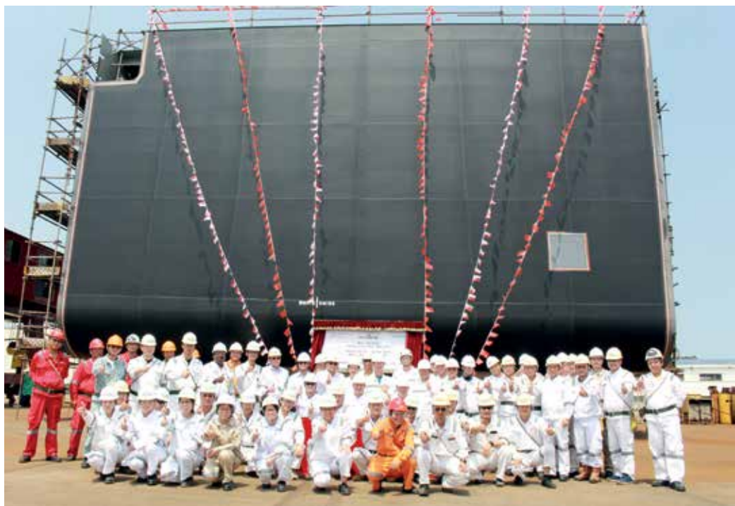
The Keppel Nantong team marked the laying of the keel for the pontoon of the first mid-water semisubmersible drilling rig being built for Awilco Drilling
